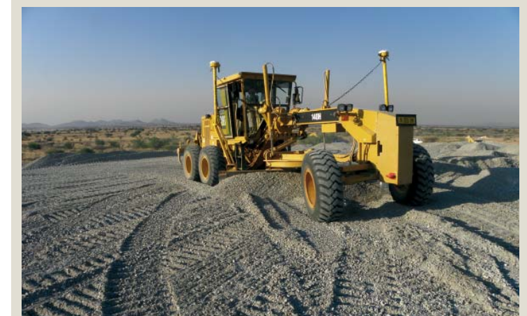
▲ The grader, now with the system fitted.
